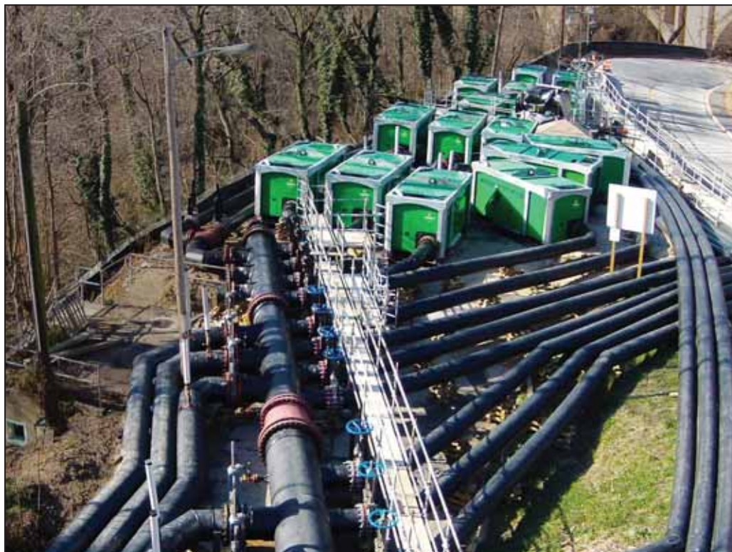
Sewer bypass completed in Baltimore, MD., with 16 18" Quiet Flow™ pumps, all designed and installed by Sunbelt Rentals Pump & Power Services.
