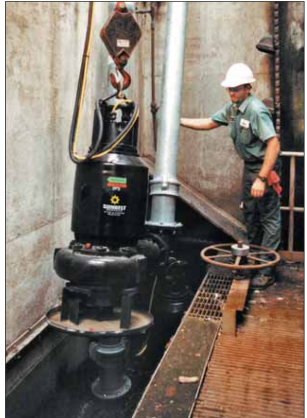
Gorman-Rupp 8" 70 HP Trash Pump One of four 8" trash pumps utilized on a wastewater treatment plant bypass job being lowered into a wet well
