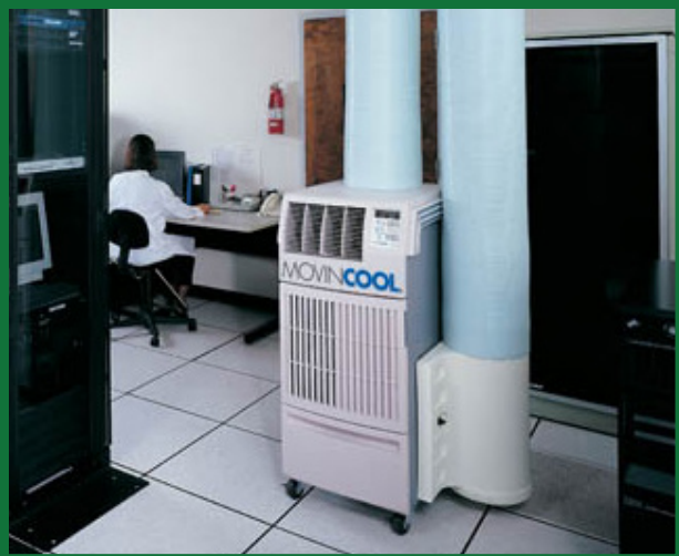
Portable units serving a large command center are hard-ducted to create an evaporator-side closed-loop system.
