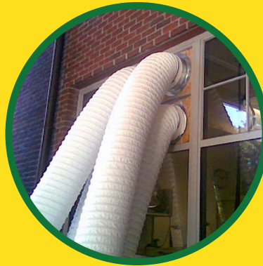
One window panel was replaced with an exact-fitting manifold with pre-cut openings for the supply and return ducts.
