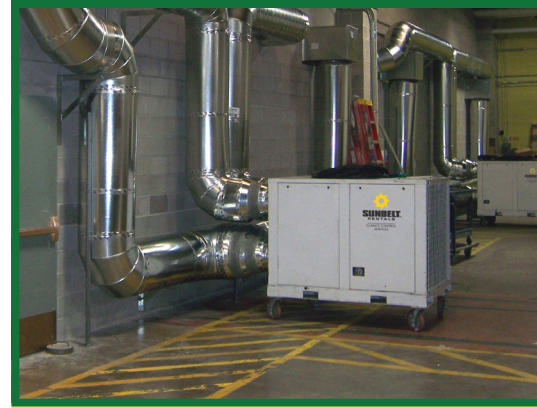
Portable units serving a large command center are hard-ducted to create an evaporator-side closed-loop system.
