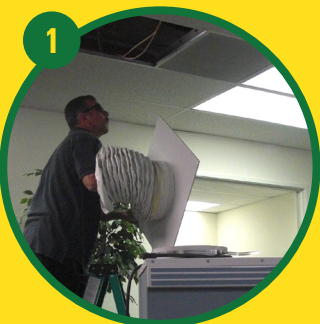
1 After removing drop ceiling tile, the technician prepares to install the ceiling exhaust kit.
