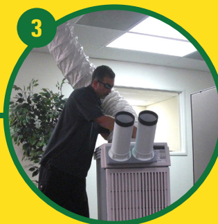
3 Portable cooling unit is wheeled into place and ducting is connected to the exhaust air vent.
