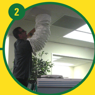
2 Exhaust duct/ceiling tile assembly is inserted directly into the opening.
