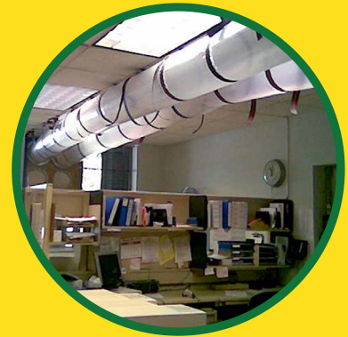
Roll-out plastic ducting was suspended from the acoustical ceiling grid, with slits at appropriate locations to maintain proper airflow.
