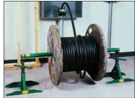
Greenlee Cable Reel Stand Set Up Two stands and one spindle are required
