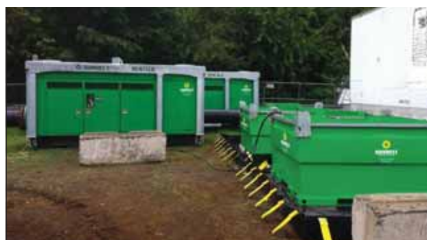
Two containment berms holding auxiliary fuel tanks at a dewatering project in Seattle, WA
