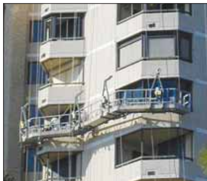
Modular staging allows unlimited versatility adapting to unusual building configurations
