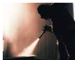
Surface Preparation Protective Coating Application
