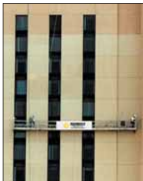
Workers using a suspended platform performing an exterior inspection at a high rise hotel
