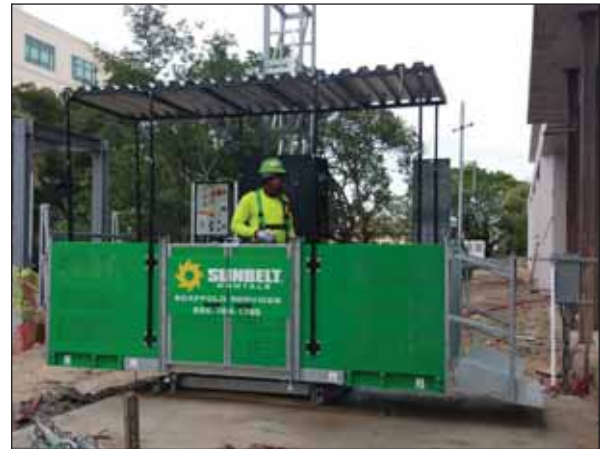
Landing gates with guard rails allow for safe and easy access to each landing
