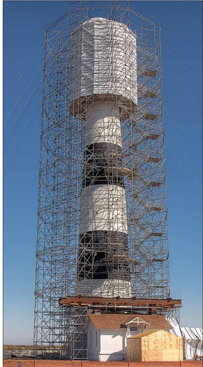
Above: Custom designed I-beams and shoring made of systems scaffold provide a clear span over the historic lighthouse's ground level oil house
