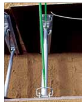
Installation and removal are performed from the top of the trench.
