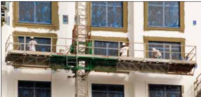
Vertical travel on mast climbers is controlled from the work platform, which allows positioning the platform at the optimum height for workers
