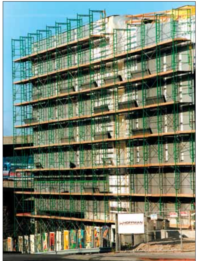
Frame scaffolding surrounding an art museum under construction
