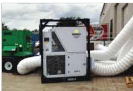
Smart Family 40-ton Industrial Air Conditioner Temporary cooling application at a warehouse facility
