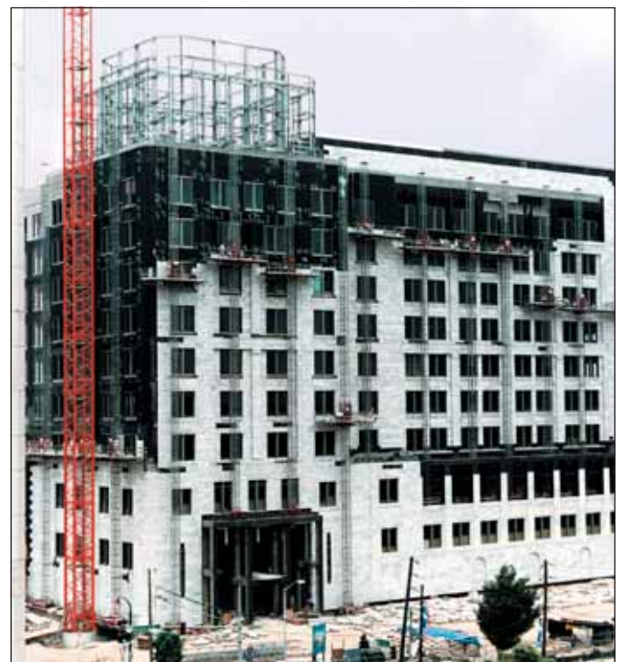
A total of 18 mast climbers were used on this project, providing access for workers installing marble on the building exterior
