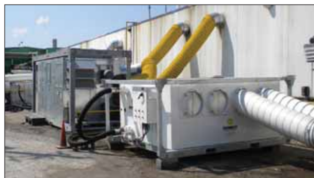
Desiccant dehumidifier and air handler at a processing plant
