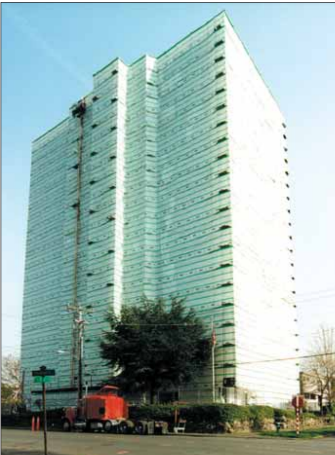
Scaffolding with a weatherproof enclosure system during the restoration of a high rise building
