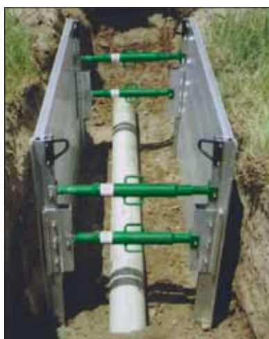
2-sided aluminum lite shield working in a pipeline application
