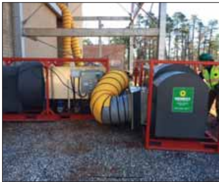
(2 Units) Safe-Heat SH-2000 400,000–2,000,000 BTU Dual Fuel Direct-Fired
