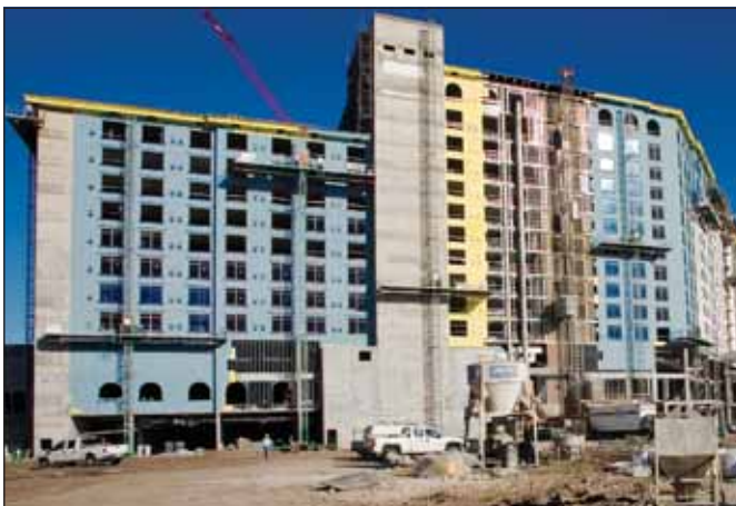
A total of 65 mast climbers were utilized during construction of this multi-sided convention hotel
