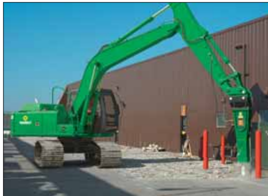
John Deere 160GLC Hydraulic Excavator w/Hydraulic Breaker
