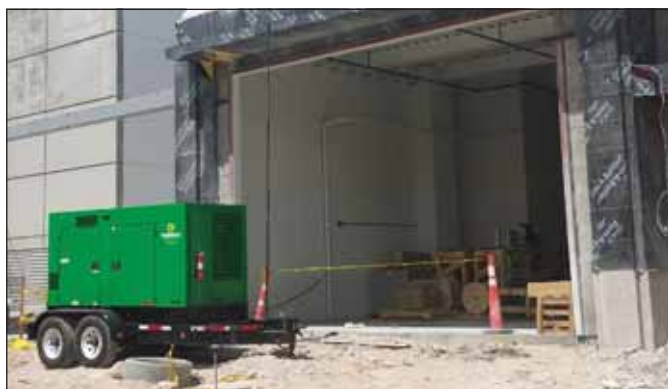
MQ Power 100 kW Towable Generator Temporary power for a construction site
