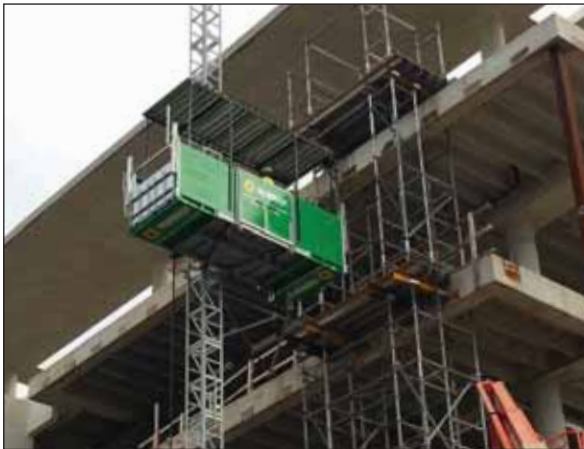
Floor stop bars allow for automatic stopping at each landing
