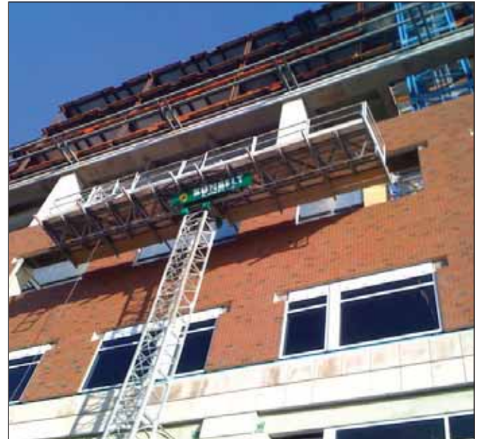
Mast climbers allow workers to install glass inserts and outer decorative panels for the entire building in a quick and efficient manner
