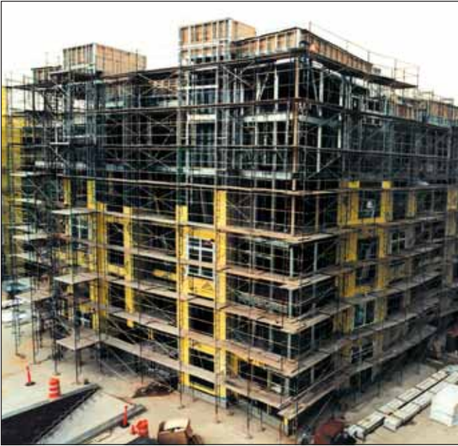
A large frame scaffold installation erected at an apartment complex under construction
