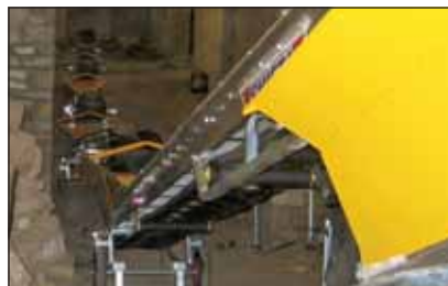
Multiple sectional conveyors working on an underground excavation project
