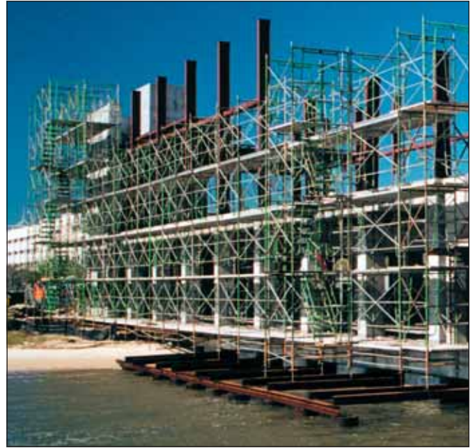
A frame scaffold installation at a new tour boat facility under construction
