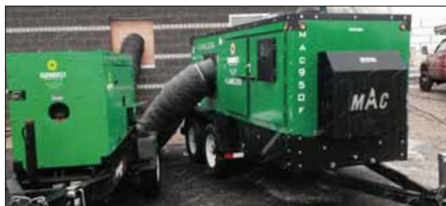
MAC 950F Flameless Heater Providing heat on a construction site
