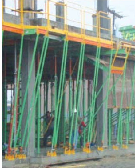
The TABLA K-Clamp connected to Tabla Deck Cantilever system to form a perimeter beam
